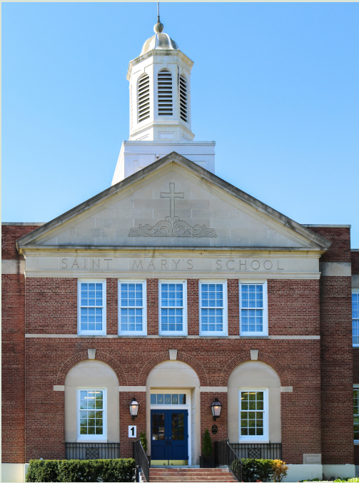
Basilica School of Saint Mary Restoration of Cupola with 1811 School Bell.
